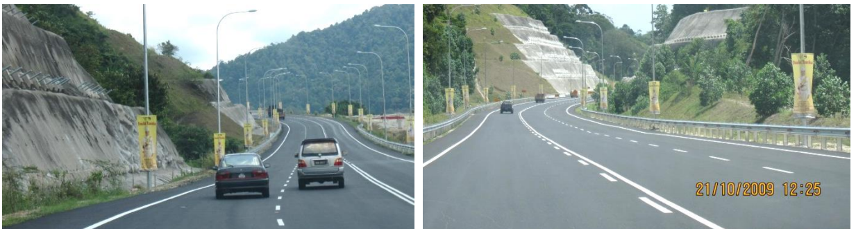
Upgrading of road from Seremban to Kuala Pilah, Negeri Sembilan (Phase 1 : Senawang Junction to Bukit Putus)
