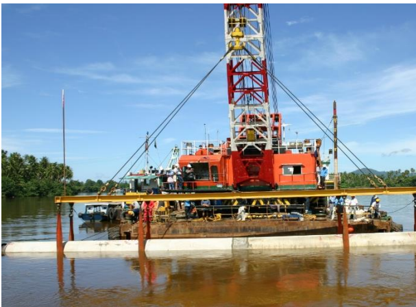
Kuala Terengganu Phase IV Water Supply Project, Top: Kepong Water Treatment Plant, Kuala Terengganu, Bottom right: Overview at Kepong Treated Water Pump House, Kuala Terengganu, Bottom left: 1,200 mm dia. Cladded Pipe Laying Work across Sg. Terengganu from Losong Feri to Bukit Datu.
