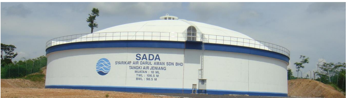
Sik Water Supply Scheme Project in the State of Kedah Top: 10 ML Jeniang Reservoir Bottom: Jeniang Water Treatment Plant
